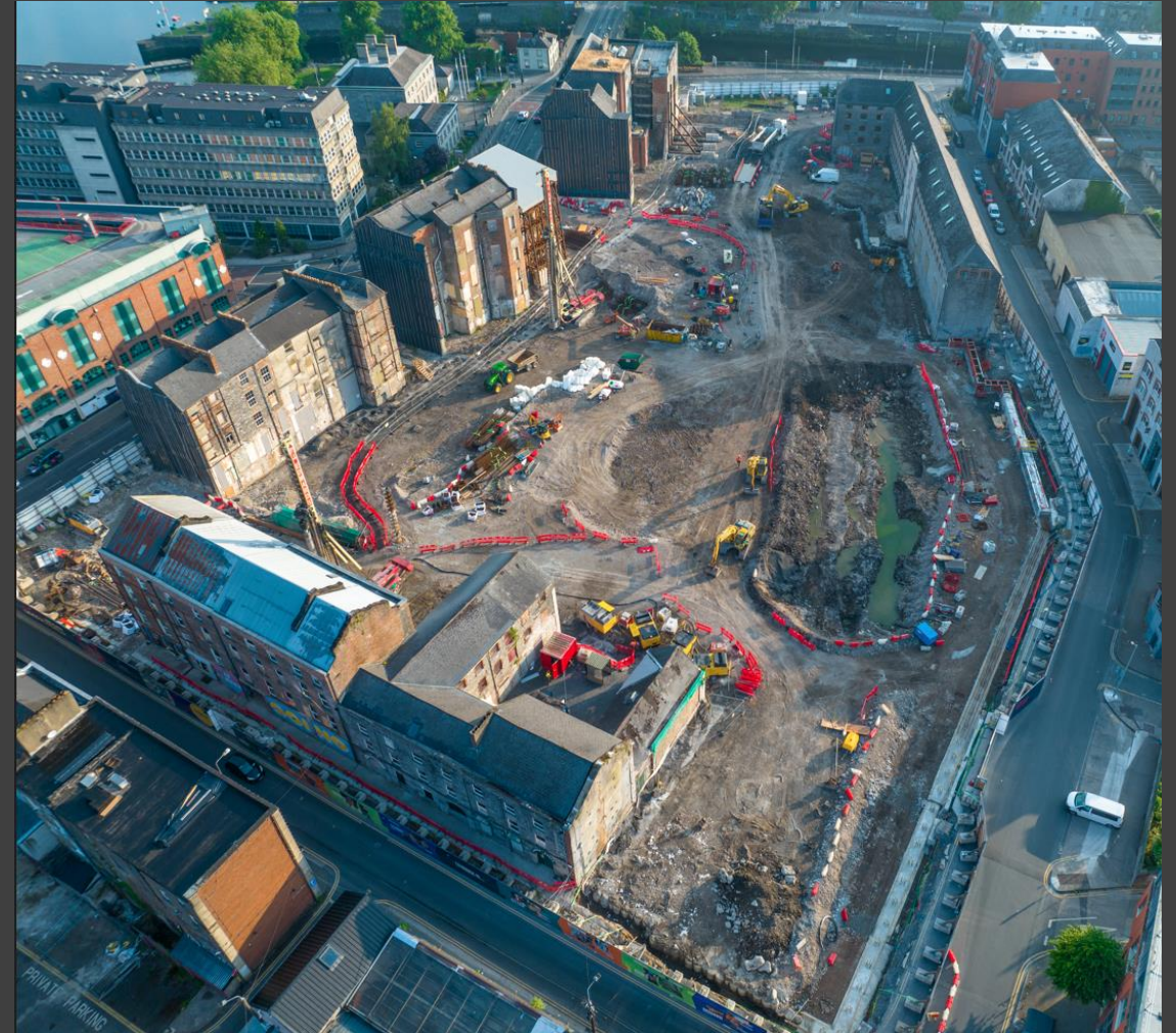
BASEMENT EXCAVATION MAY 2023
