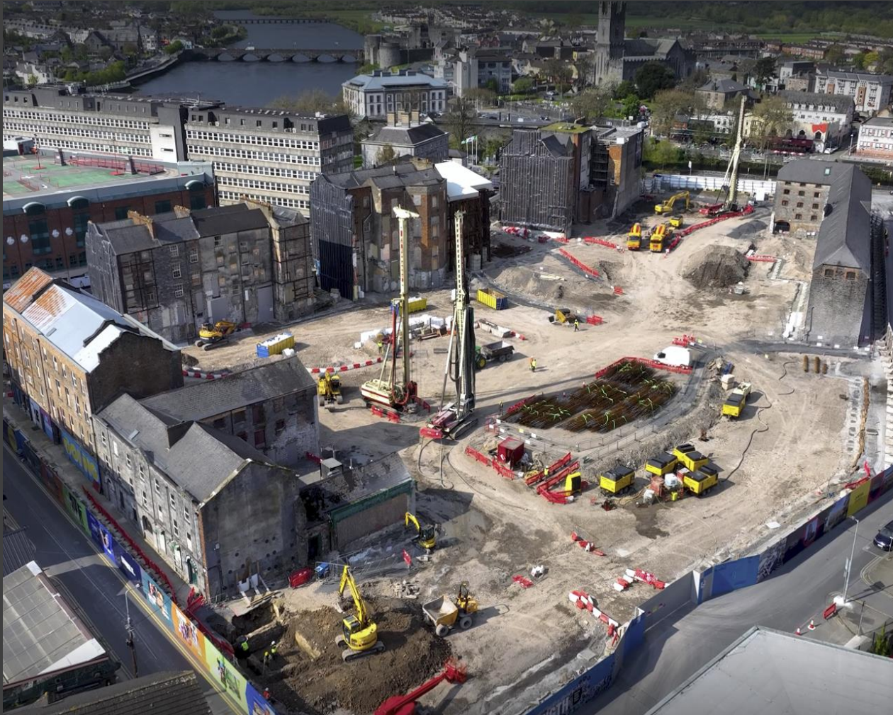
PILING WORKS MARCH 2023
