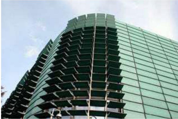
Nordic Embassies, Berlin Green Cladding wall louvres motion Courtesy of Lucas Gray, talkitect.com, 2008
