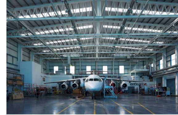
City Jet Aircraft Hangar €6.6 million
