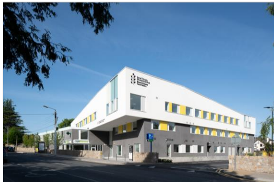
Bray Primary Care Centre Confidential
