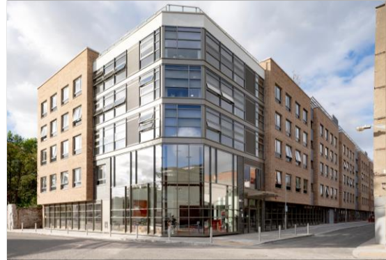
Brickfield Lane Student Accommodation €19.6m
