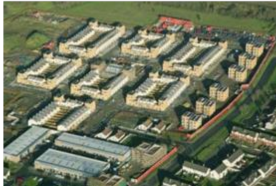
232 Units, Tyrellstown €48.8m
