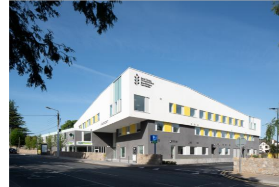
Bray Primary Care Centre Confidential
