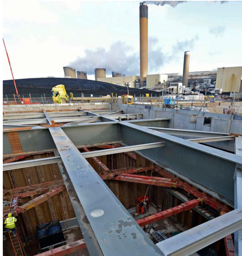
Cofferdam installation
