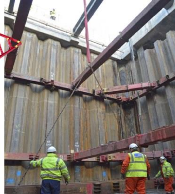
Cofferdam installation
