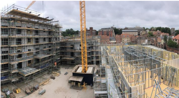
Figure 2: erection of 2D Smart Modular Elements
