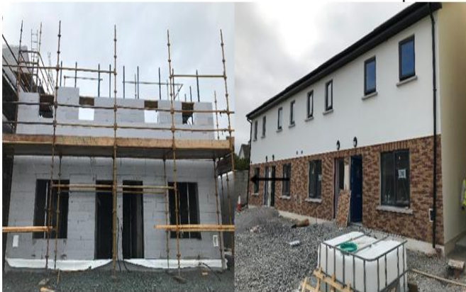
Figure 3: Initial arrival onsite through to completion.
