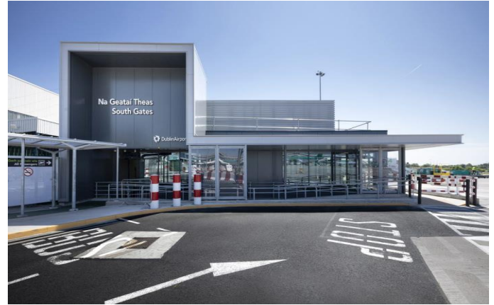
Figure 3 – South Gates Dublin Airport
