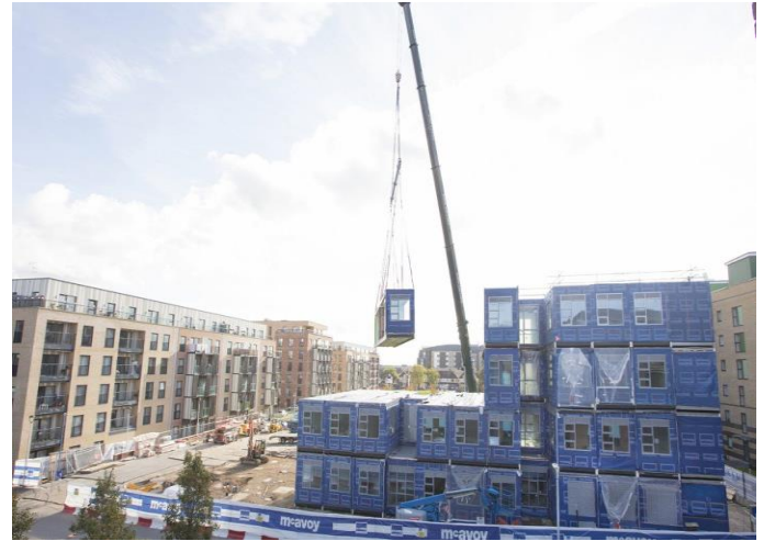
Figure 2 – Building craned into position
