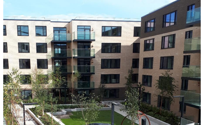
Progress photo of Block B/C Courtyard
