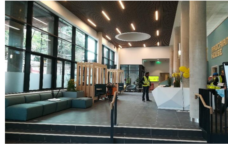
Progress photo of Entrance area
